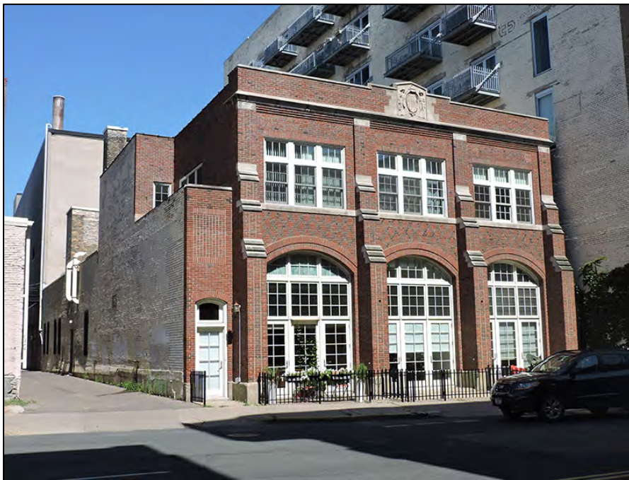
Figure 26. Engine House No. 2 at 412 North Wacouta Street, 2016
