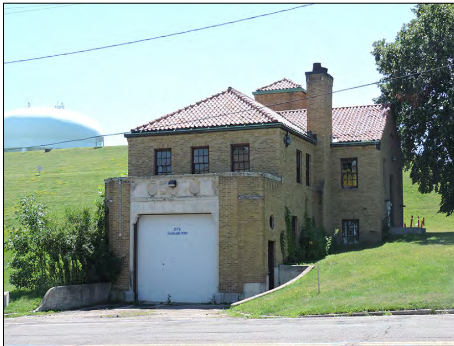
Figure 25. Engine House No. 19 at 750 Snelling Avenue South, 2016
