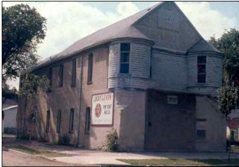
Figure 11. Station 12 at 700 Jackson Street NE, n.d. 57
