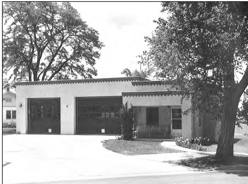
Figure 9. Fire Station 2, Albuquerque, New Mexico, built 1937 46
