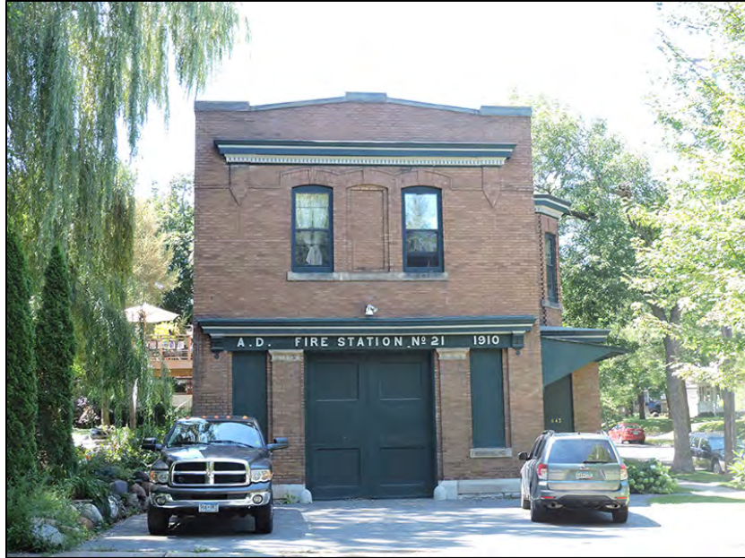
Figure 23. Engine House No. 21 at 643 South Ohio Street, 2016
